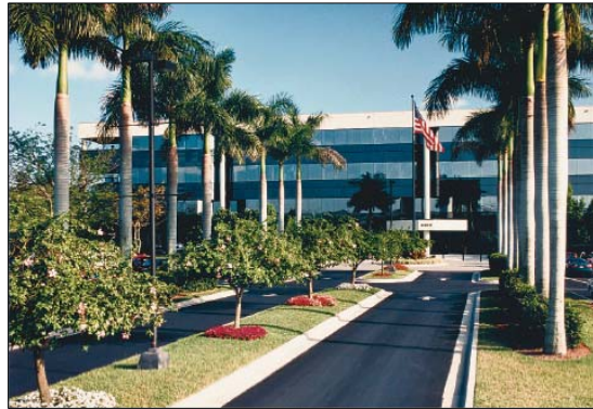
Doral's new City Hall and Police Station is located at 8300 NW 53 Street.
