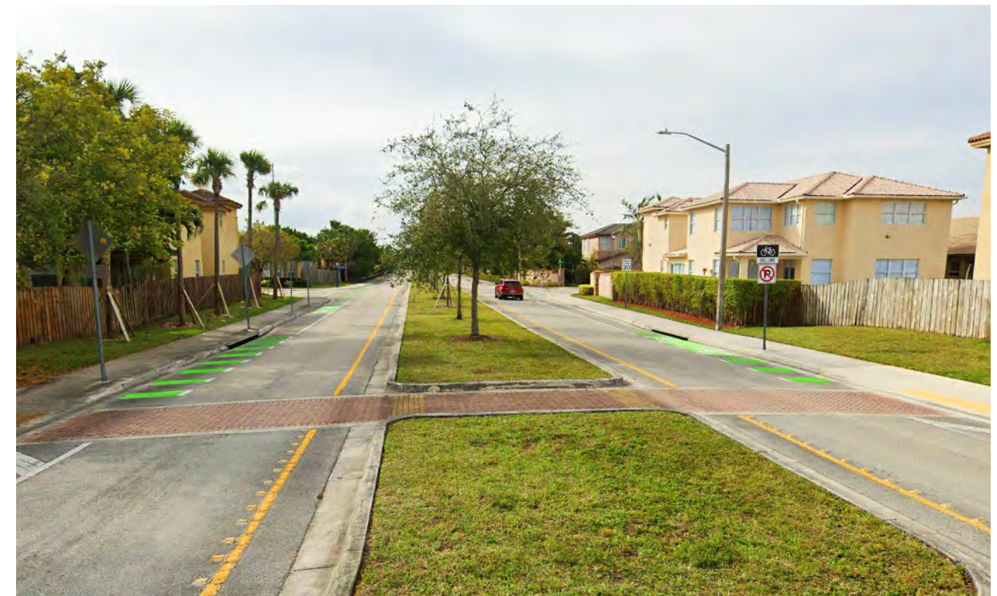
Figure 3-4: High Visibility Bicycle Lanes - NW 112 th Avenue between NW 74 th Street and NW 82 nd Court
