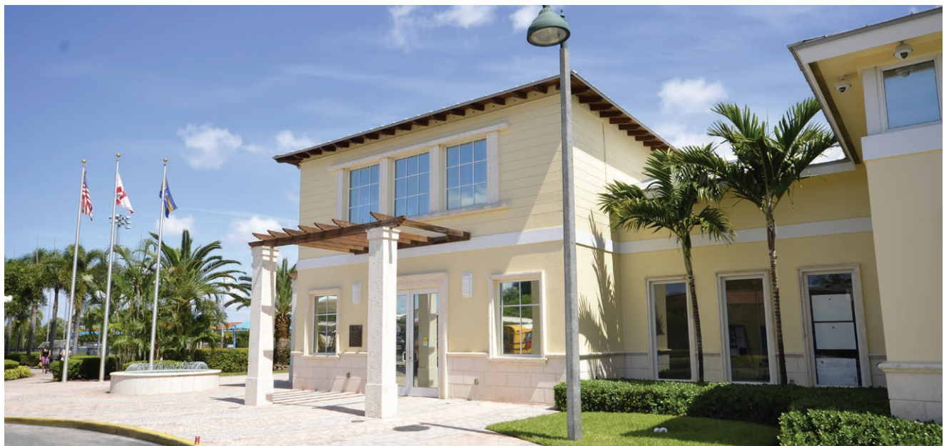
Figure 5.2: Morgan Levy Community Center that is recommended for future expansion to 15,000 SF.
