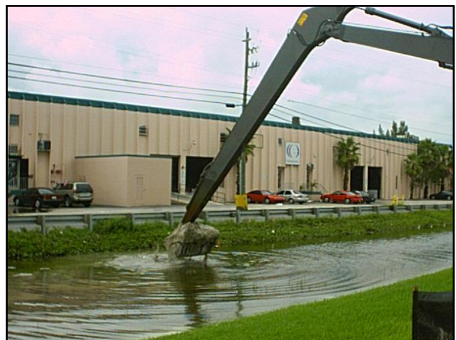
Canal Cleaning & Shaping
