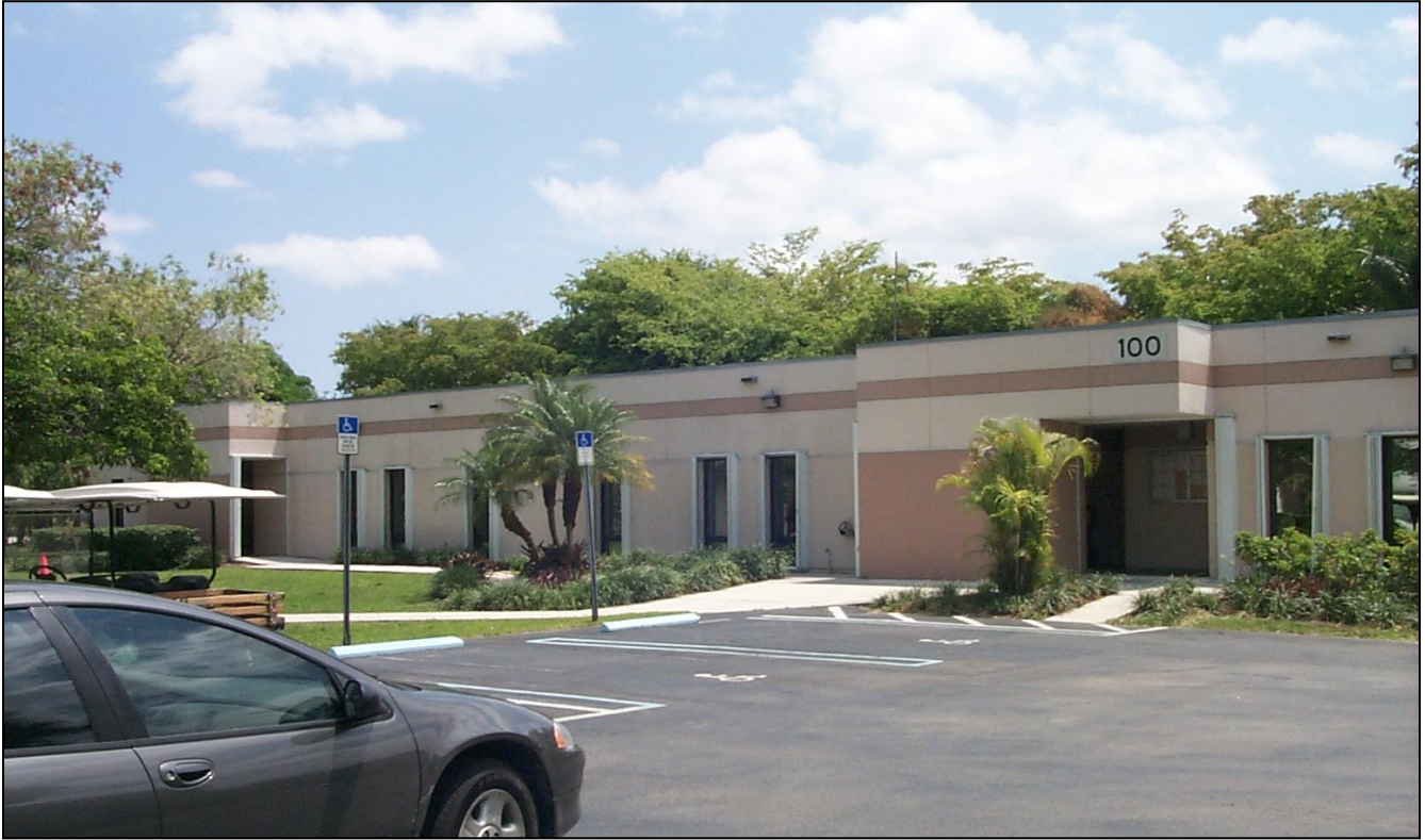
The Miami-Dade Police Training Bureau building was hardened at a cost of $102,000 funded by the Hazard Mitigation Grant Program through FEMA-1545-DR-FL
