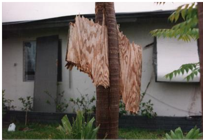
Damage showing impact of Hurricane speed winds
