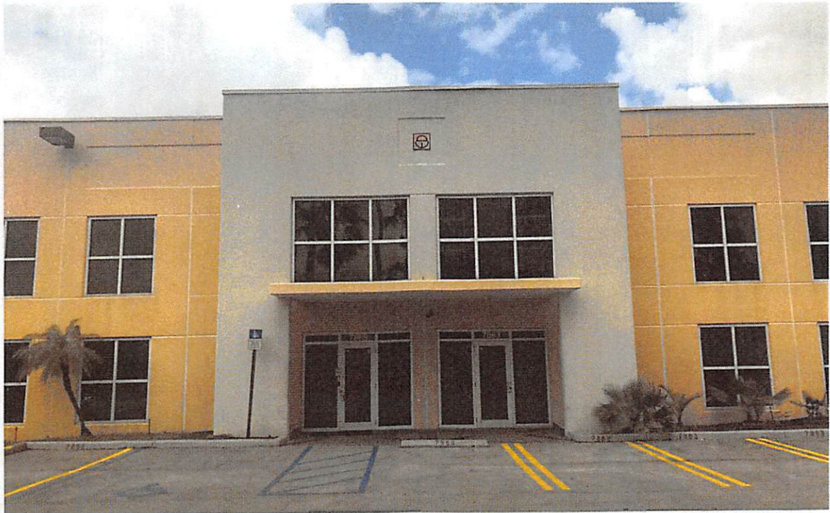
CURRENT BUILDING FACADE
