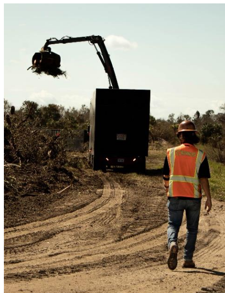
Ceres collected over 2.4 million cubic yards of Hurricane Ian debris in the City of North Port, FL alone
