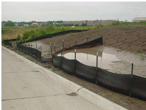
Figure 10-3 – Stacked Turbidity Barrier or Silt Fence (c)
