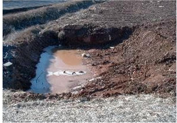
Figure 10-4 – Sediment Trap & Spillway
