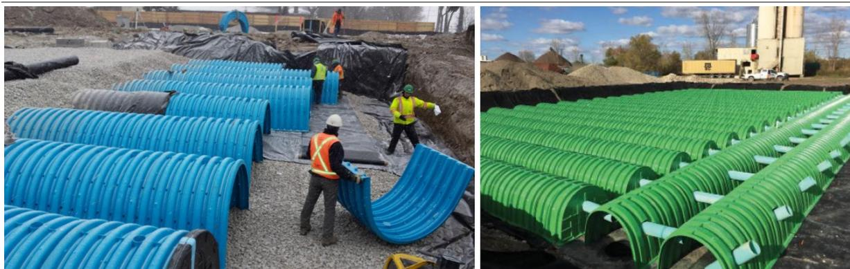
Figure 6-24 – Stormwater Chambers
