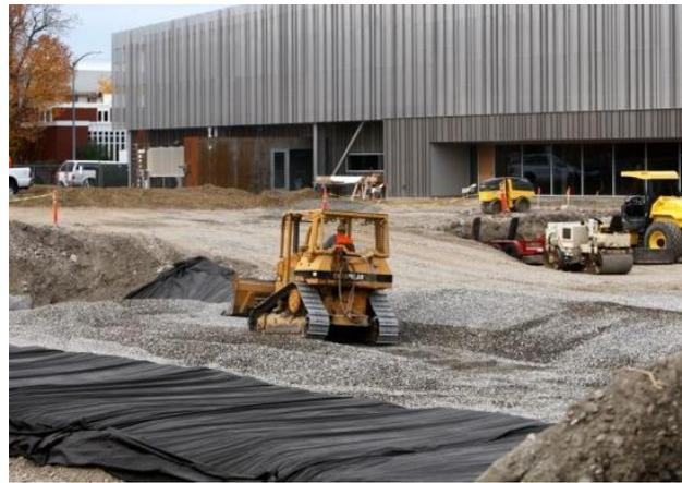
Figure 10-1 – Temporary Gravel Construction Entrance & Exit (a)
