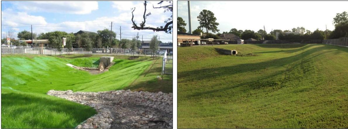
Figure 6-21 – Typical Dry Retention Pond
