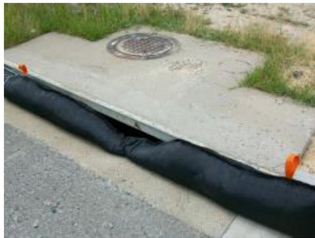
Figure 10-2 – Storm Drain Inlet Protection (b)
