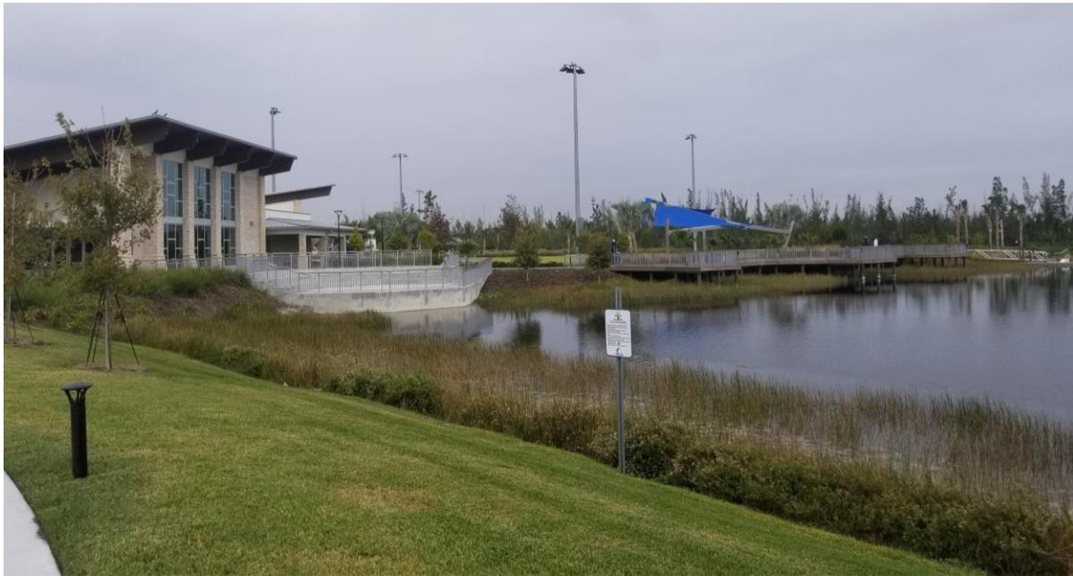
Figure 6-22 – Doral Glades Park Stormwater Wet Retention Pond
