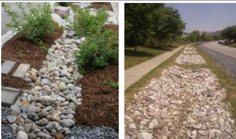
Figure 6-11 – Infiltration Trench
