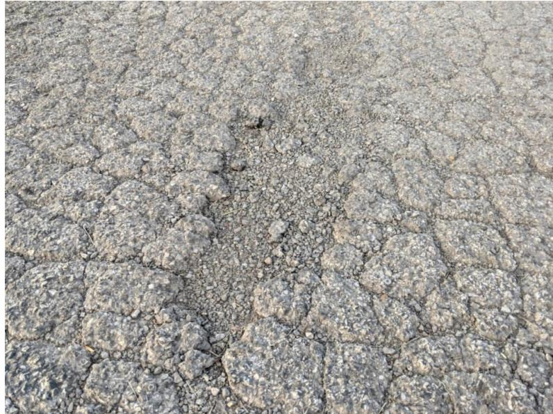
***Figure 8. Pavement showing severe raveling***
