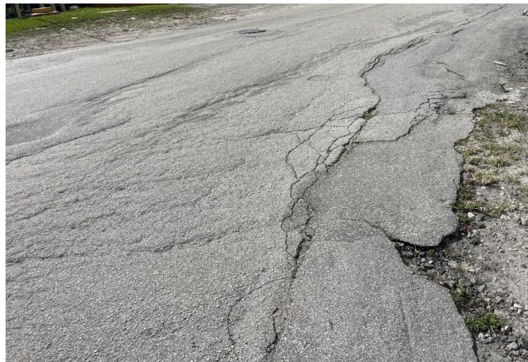
*Figure 7. Advanced rutting with severe pavement displacement*
