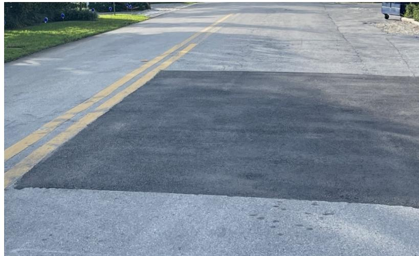
**Figure 12. Roadways showing pavement patching**
