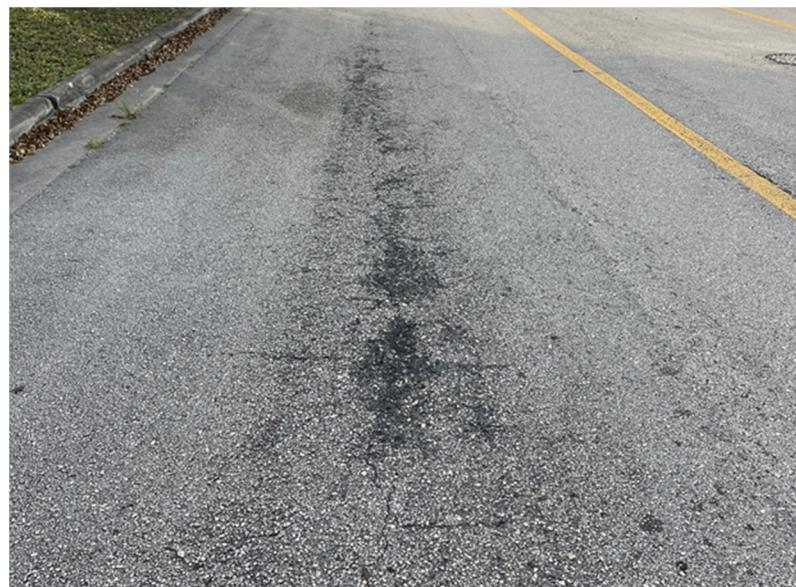
***Figure 9. Pavement showing moderate raveling***
