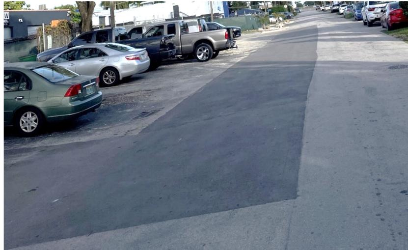
**Figure 11. Longitudinal patching on pavement**
