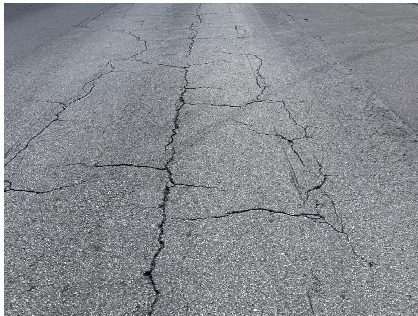
*Figure 3. Class III crack, extend in a longitudinal direction*
