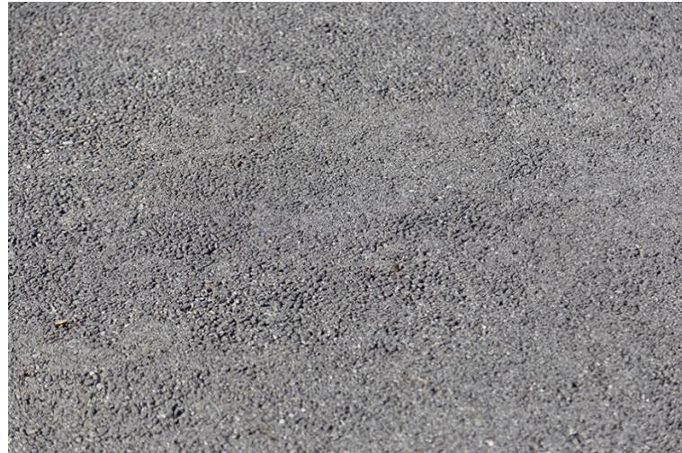
**Figure 10. Pavement showing light raveling**
