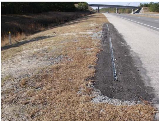
Figure 4. Edge-of-pavement slot drain.
