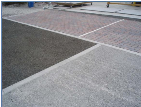
Figure 1 Pervious Pavement Sections at the UCF Research Facility
