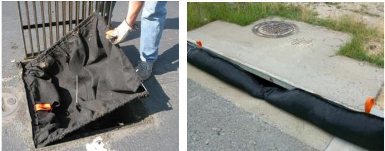
Figure 10-2 – Storm Drain Inlet Protection (b)
