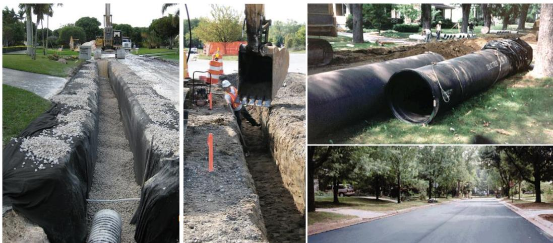
Figure 6-13 – Exfiltration Trench
