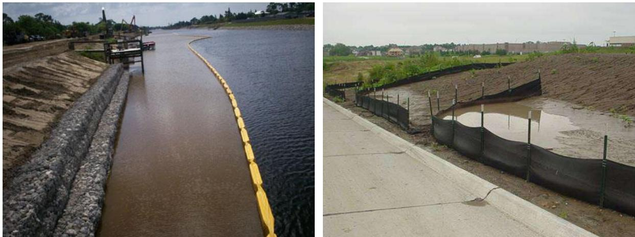
Figure 10-3 – Stacked Turbidity Barrier or Silt Fence (c)
