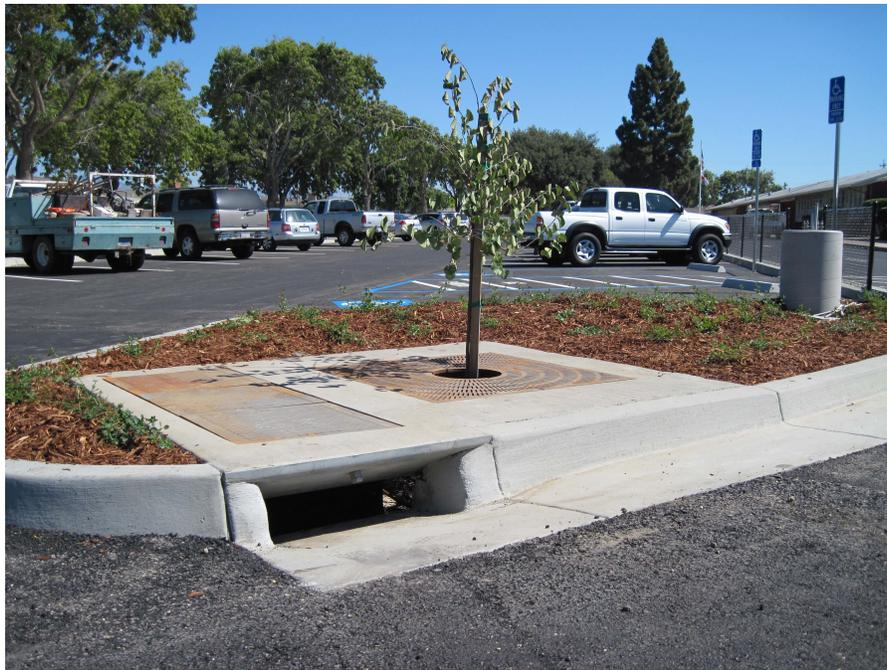
**Figure 12 - Newly Installed Urban Green BioFilter**
