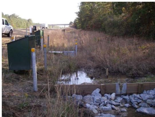
Figure 8. Outlet structure for swales.
