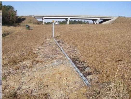
Figure 5. Downslope edge of filter strip slot drain.
