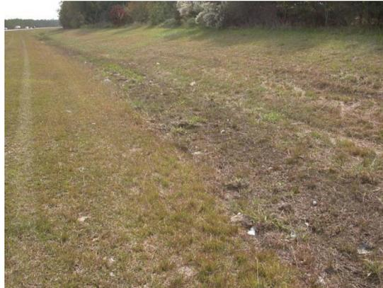
Figure 2 Example of a vegetated swale without wetland characteristics (i.e. standard dry swale).
