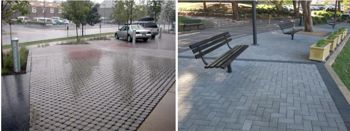
Figure 6-19 – Permeable Pavement in Parking Lot and Park/Walkaway Area
