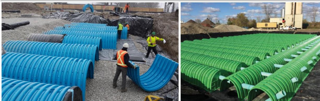
Figure 6-24 – Stormwater Chambers
