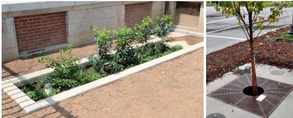
Figure 6-4 – Infiltration Planter and Tree Box
