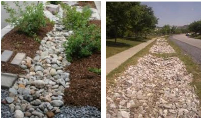
Figure 6-11 – Infiltration Trench
