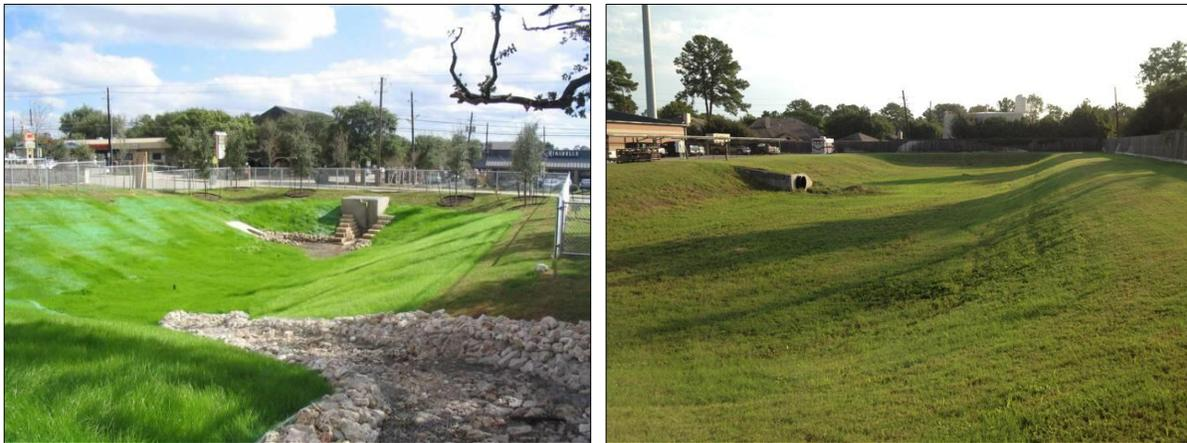
Figure 6-21 – Typical Dry Retention Pond
