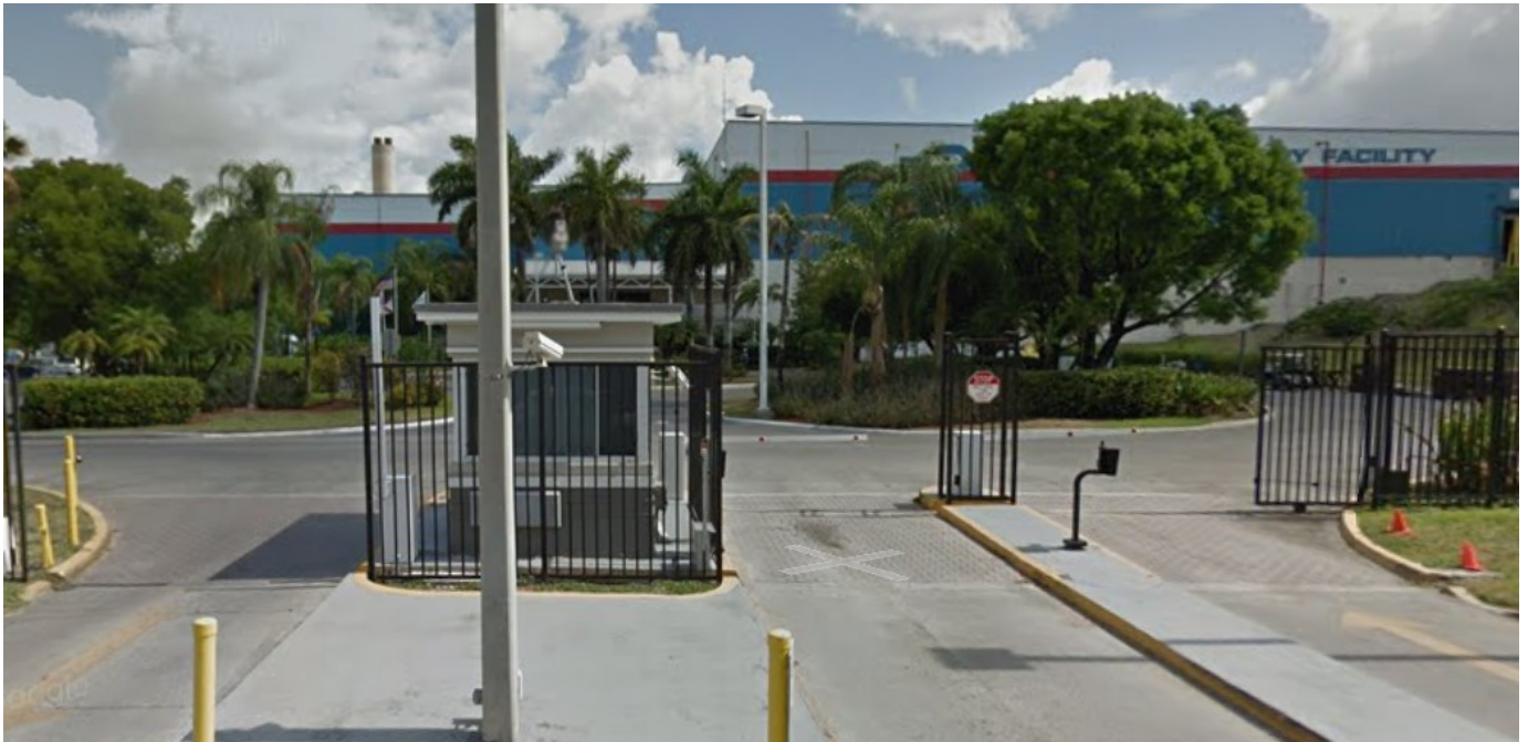
Resources Recovery Facility – NW 66 th Street (Source: Google Maps)
